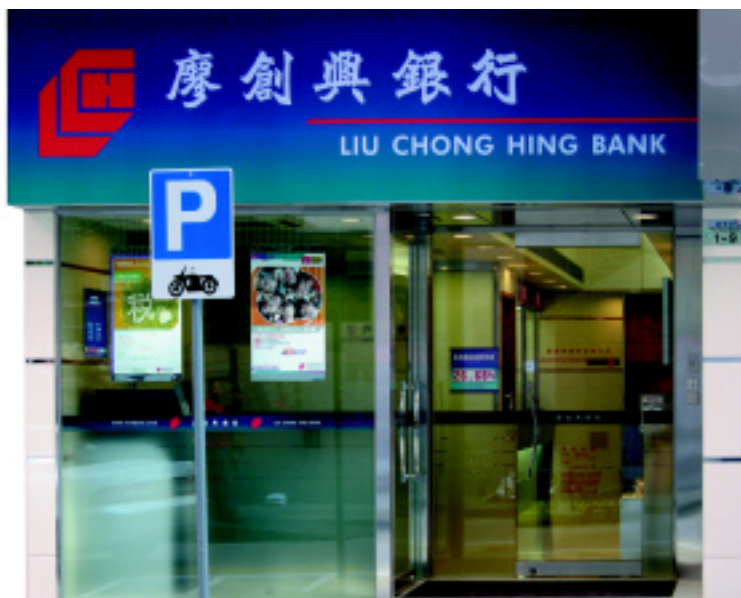
New face of Happy Valley Branch after renovation
